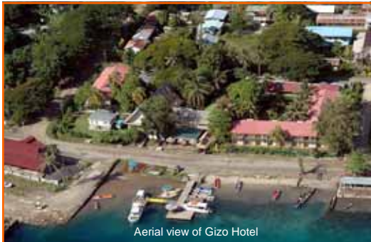
Aerial view of Gizo Hotel
